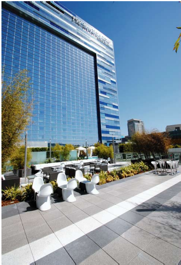
Above & Left Photos: LA Live Ritz Carlton / JW Marriott; Architect: Gensler; Finish: GraniteTech; Size & Color: 20" x 20" Charcoal, Gray Black & White Black; Application: Roof Deck - Pedestal Set
